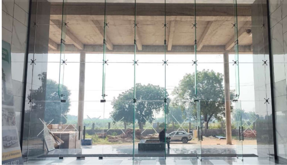
COMMERCIAL PROJECT – STRUCTURAL GLAZING
